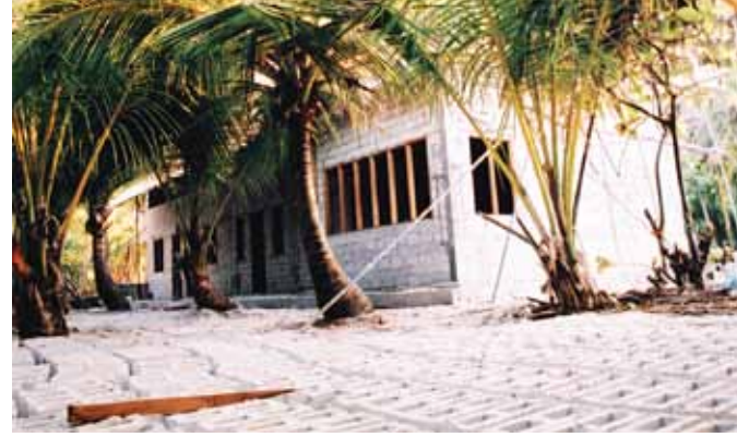
Casting blocks from the beach sand and senior staff house.
