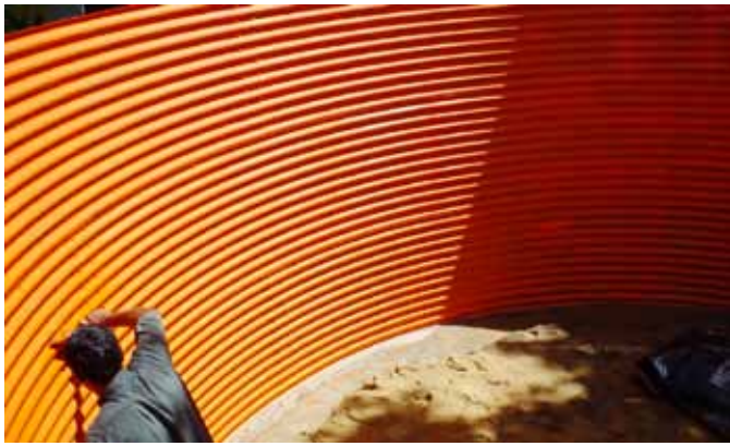
Installation of 60m 3 watertank.
