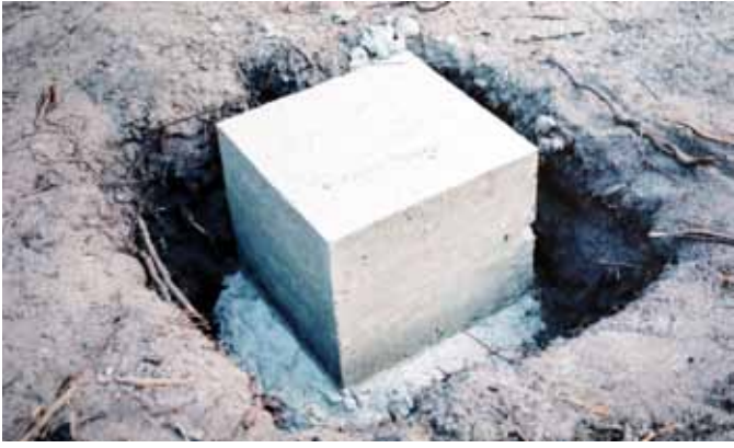
Shadehouse foundation block.
